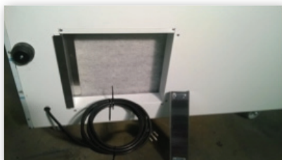
Slide off the filter locating brackets
