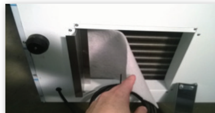
Remove old filter and fit new filter in reverse
